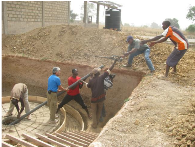
Figure 35: Raising center pole
