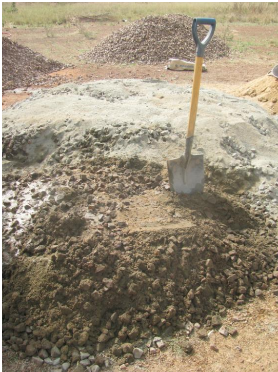
Figure 41: Pile of cement, sand, and aggregate (1:2:4 ratio) ready for manual mixing
