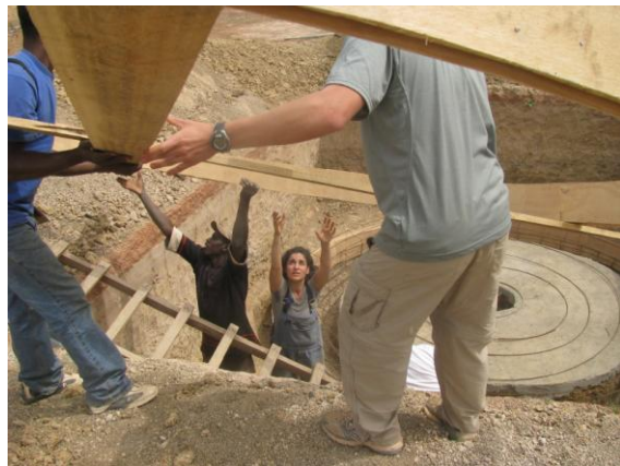
Figure 34: Lowering the inner form
