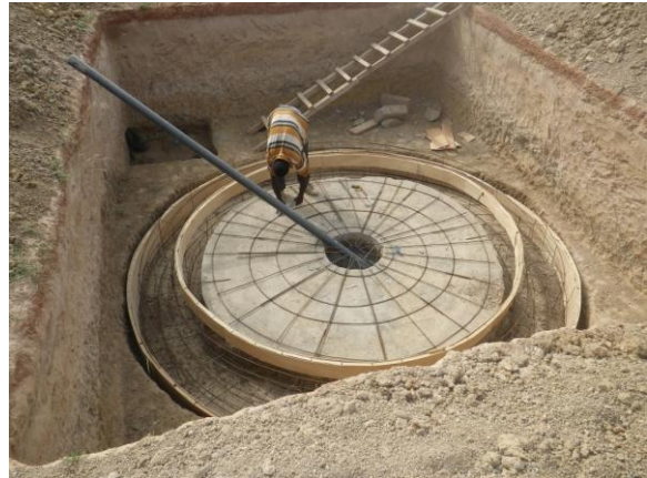
Figure 25: The steel bender links reinforcement for tank floor with reinforcement for footing
