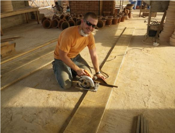
Figure 27: Mitch Westwood kerfs planks of wood for the formwork
