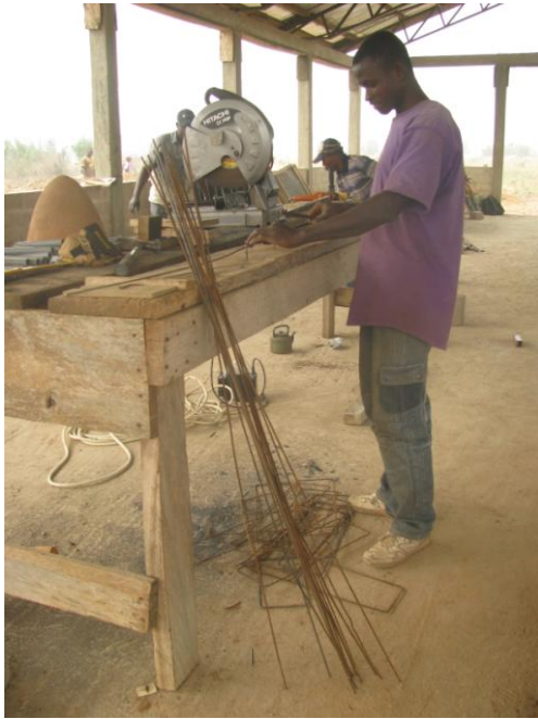
Figure 20: The steel bender bending 1/2 inch rebar
