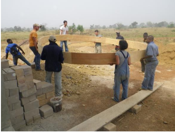
Figure 31: Carrying the outer form over to the excavated site
