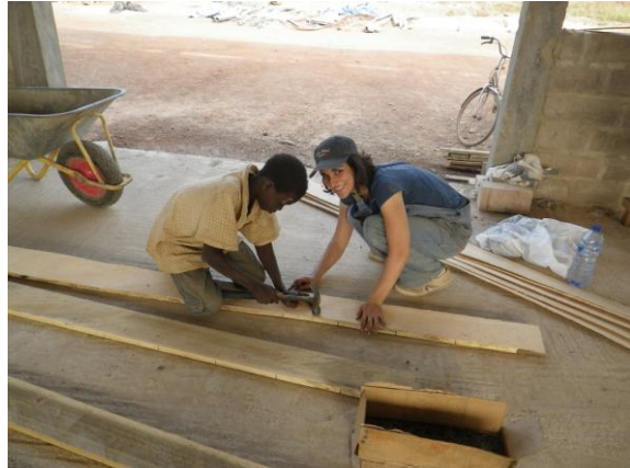
Figure 28: Shanti Kleiman and Zachary nail plywood to the kerfed boards
