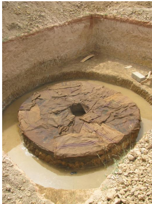
Figure 19: This layer was kept moist with wet burlap bags for two days while it dried
