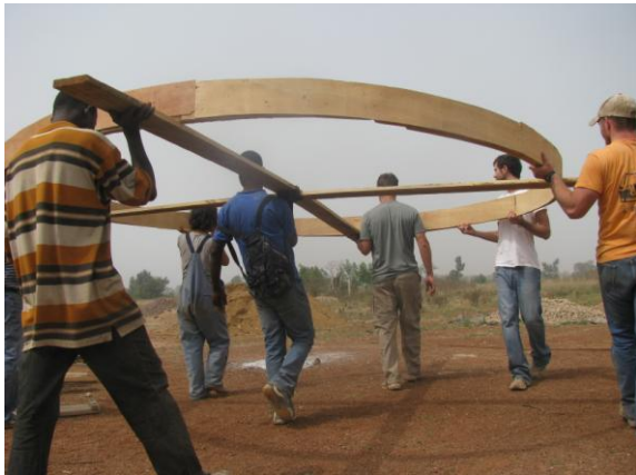
Figure 33: Carrying the inner form
