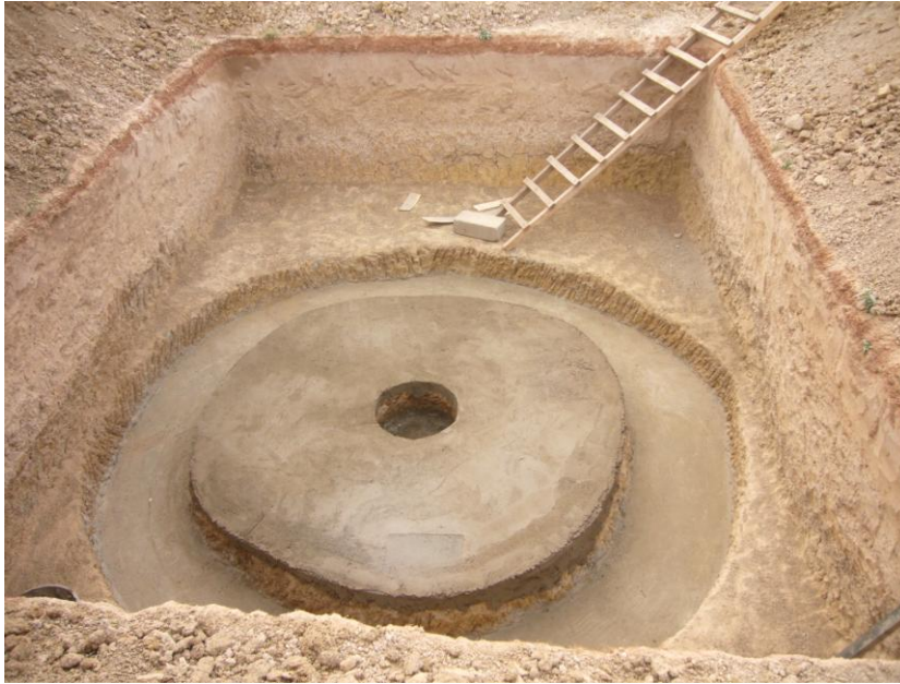
Figure 18: 2-inch base layer applied
