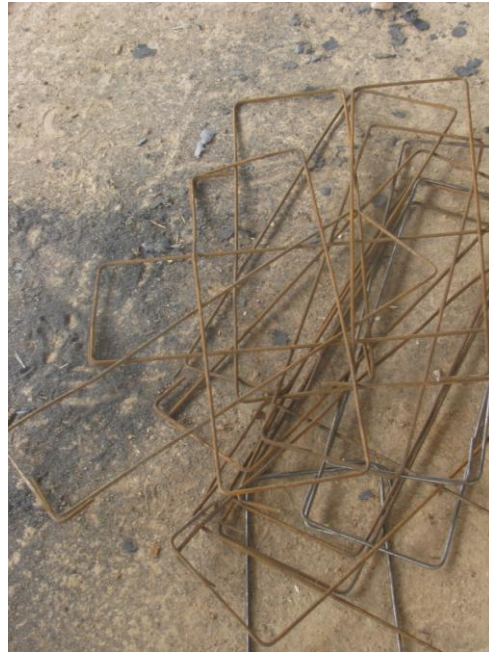
Figure 21: Close up of rectangular pieces that binds concentric circles of rebar together for the footing
