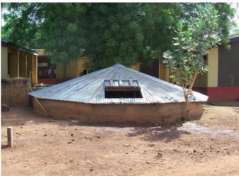
Figure 9: Service Access (Barnes 2009)
