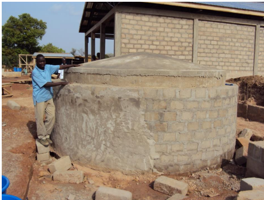
Figure 48: Post-January work: Tank walls are plastered with stucco
