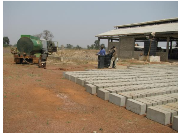
Figure 40: Water is delivered for mixing the cement for the foundation
