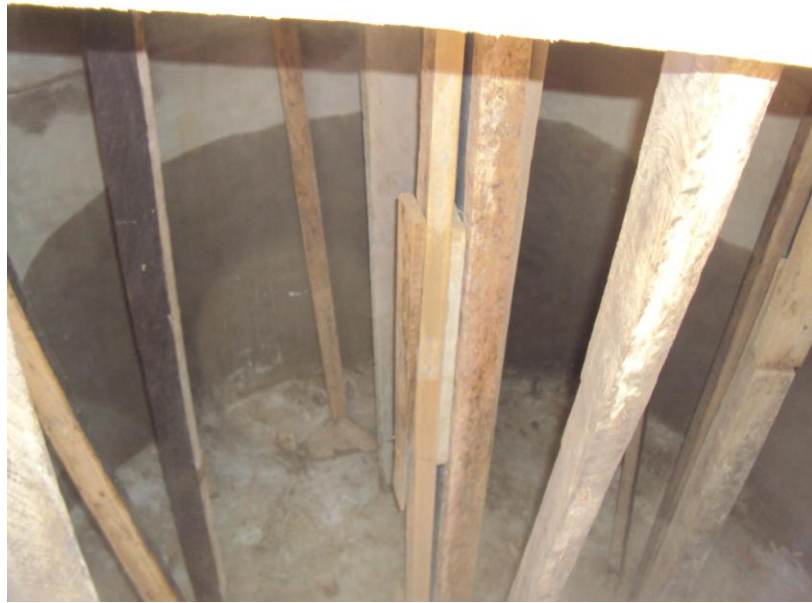
Figure 47: Post-January work: Wooden roof supports inside of tank
