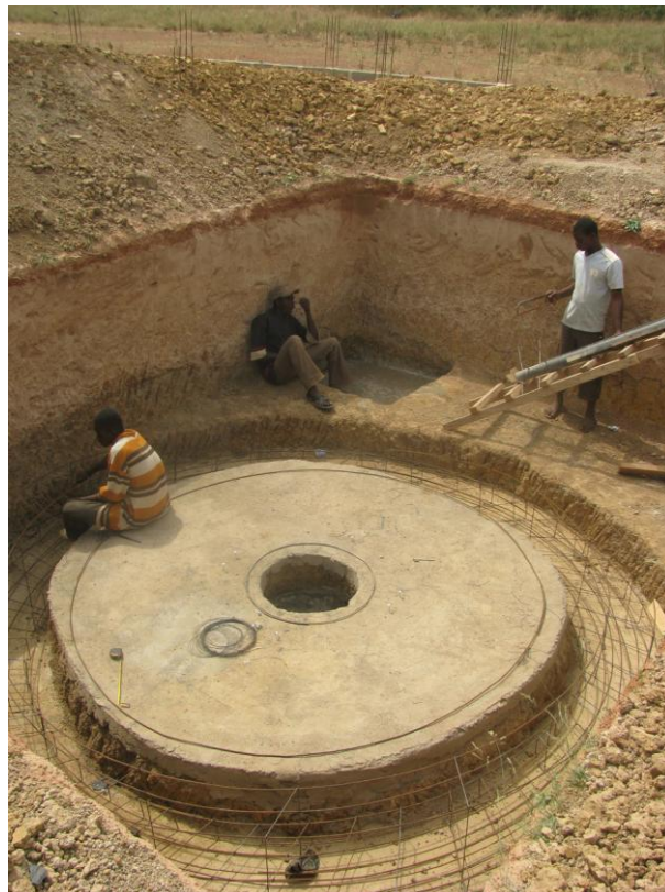
Figure 26: The steel bender begins radial reinforcement
