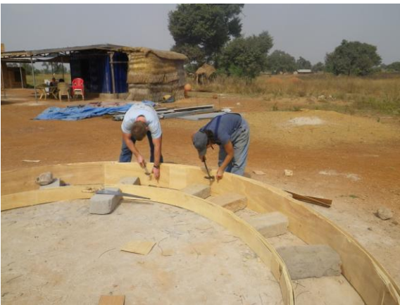
Figure 29: Shanti Kleiman and Mitch Westwood patch up the circular forms after bending the wood into a circle
