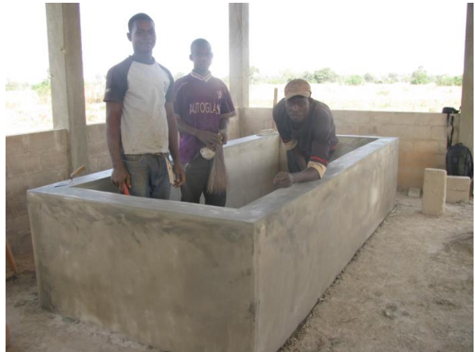
Figure 54: Sadat, Alhassan, and Shani stand inside of the completed tank
