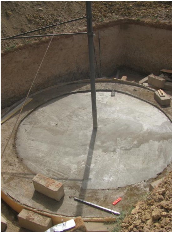
Figure 45: Finished Foundation
