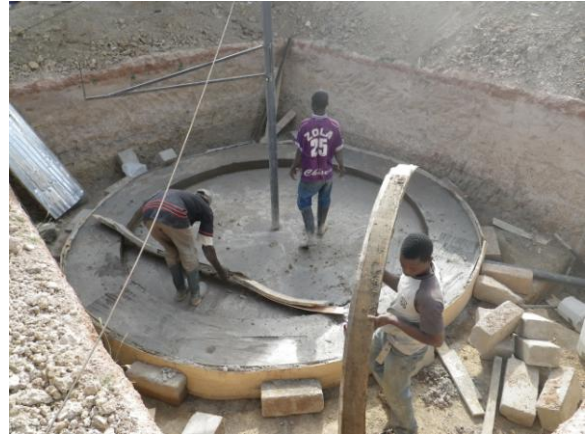
Figure 44: The forms are removed the next day
