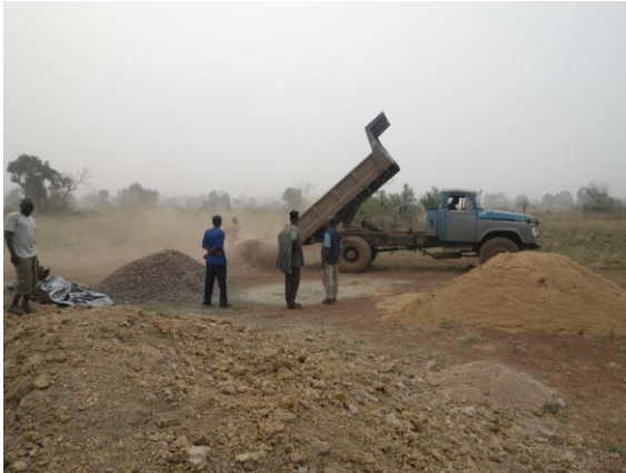
Figure 39: Stone chips are delivered for use in the foundation cement mixture
